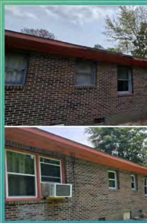
New windows (seen in bottom photo) and exterior doors were installed.
