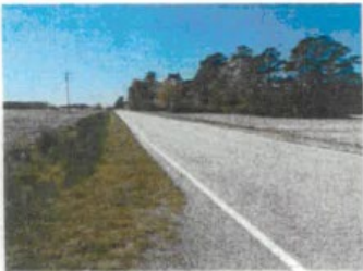
8. Road frontage to the south
