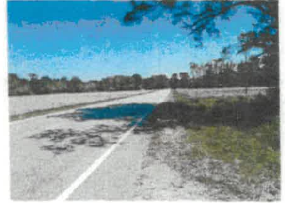
9. Road frontage to the north
